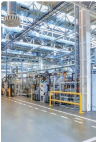
Industrial production energy storage
