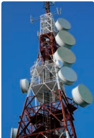
Communication base station energy storage
